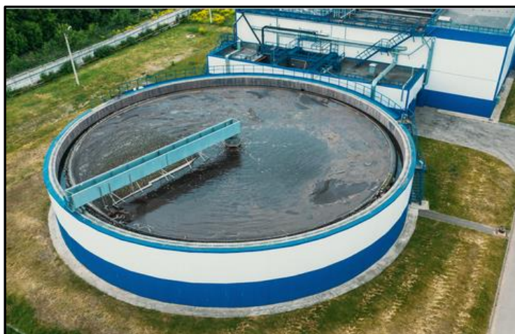
Water treatment plant with a round cylinder clarifier sedimentation tank. In sedimentation, a water treatment plant will use a clarifier sedimentation tank for removing material from liquid waste. (Mityay, n.d.)
